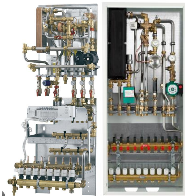
Figure 2-1b Examples of consumer substations for an individual residence with integrated heating manifolds (Photo: Danfoss and PEWO)
